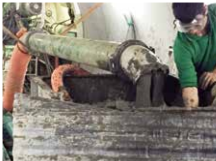
Excavated material is mixed with additive material and become plastic consistency.
