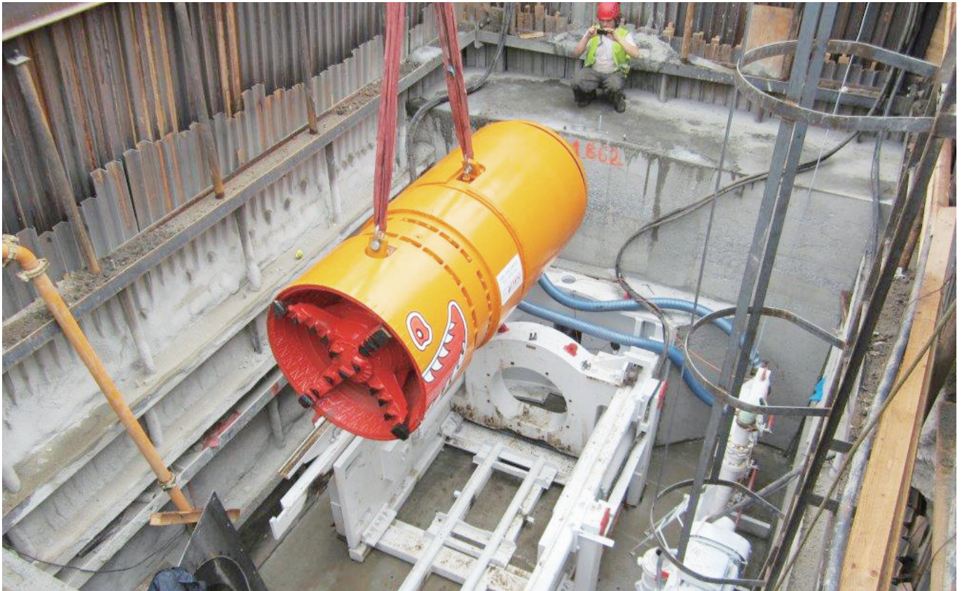
Unclemole lowering down to shaft
